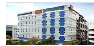
4 C&P Changi Districentre 5 5 Changi South Lane
