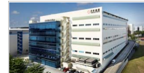
7 Hi-Speed Logistics 40 ALPS Avenue
