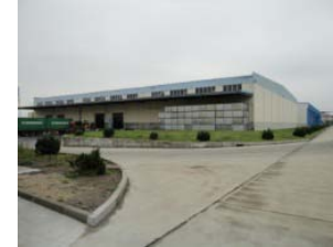
Jinshan Chemical Warehouse
