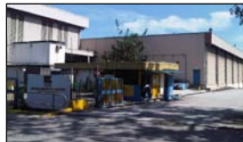
3 Kim Heng Warehouse 4 Penjuru Lane
