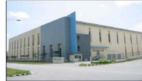
9 APC Distrihub 6 Changi North Way
